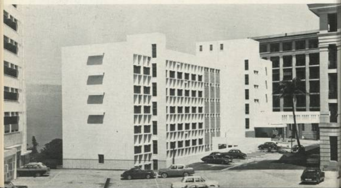
The new block housing Professorial Suites and Radiotherapy Department at Queen Mary Hospital. The bridge, at right, connects with the main Hospital building.
