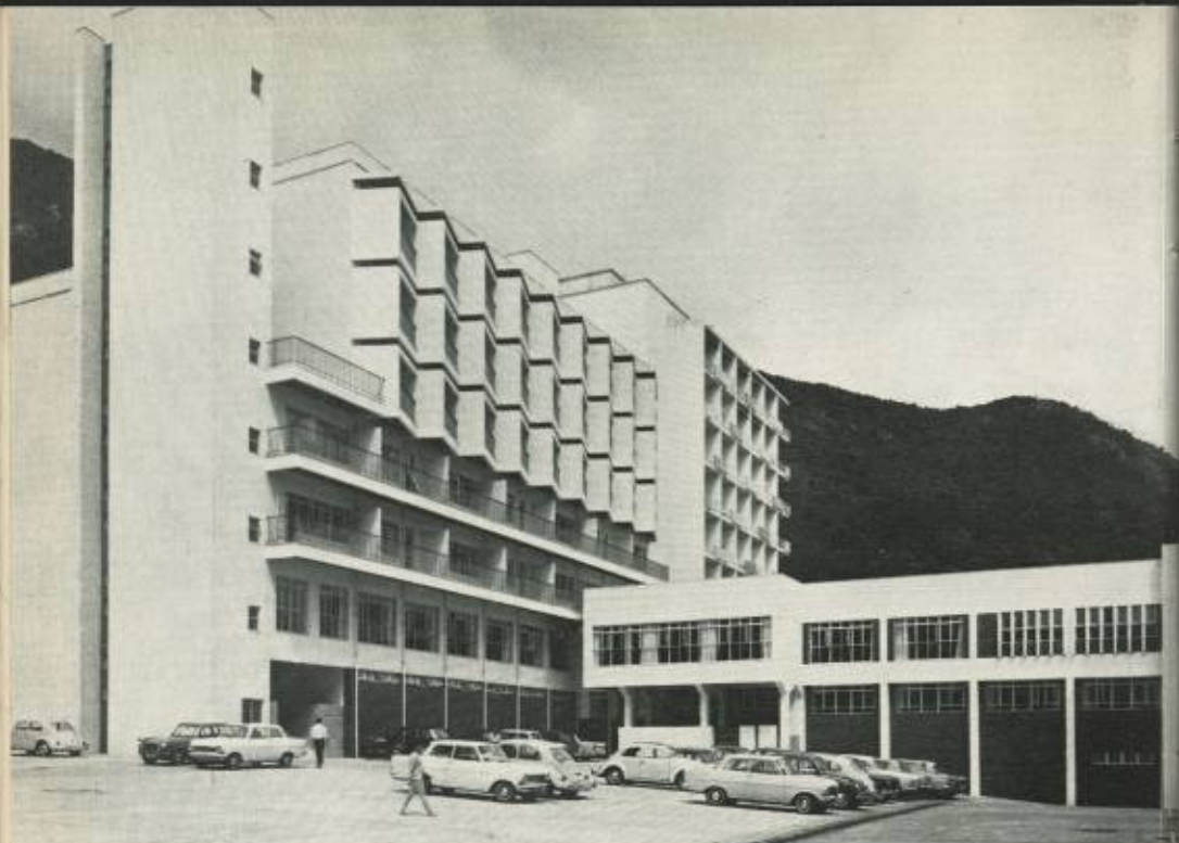
New accommodation for House Officers and Male Nurses at Queen Mary Hospital. The new Nurses Training School is seen at right of the photograph.
