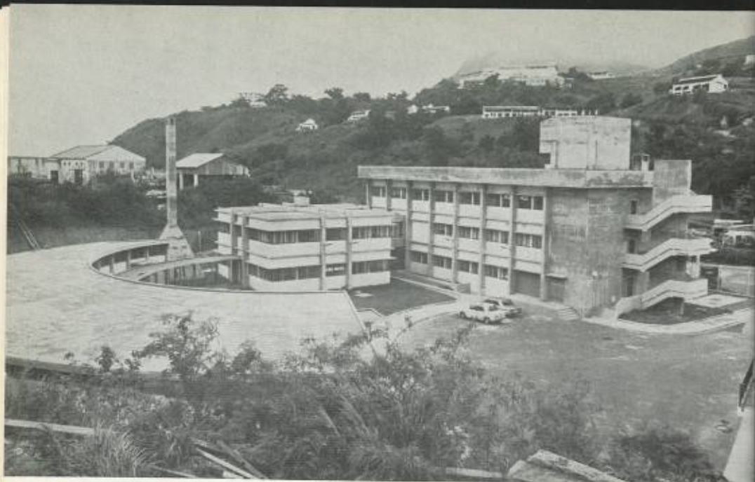
The Department's new Institute of Immunology was opened during the year, replacing the former Vaccine Institute in Caine Lane. Picture shows the series of buildings making up the Institute in a rural setting at Pokfulam.
