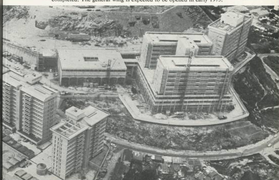
Construction of the new Princess Margaret Hospital at Lai Chi Kok progressed satisfactorily during the year. The picture above shows a section of the complex already completed. The general wing is expected to be opened in early 1975.
